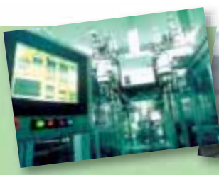
NJCTT’s production plant for PVC-free large volume injections
